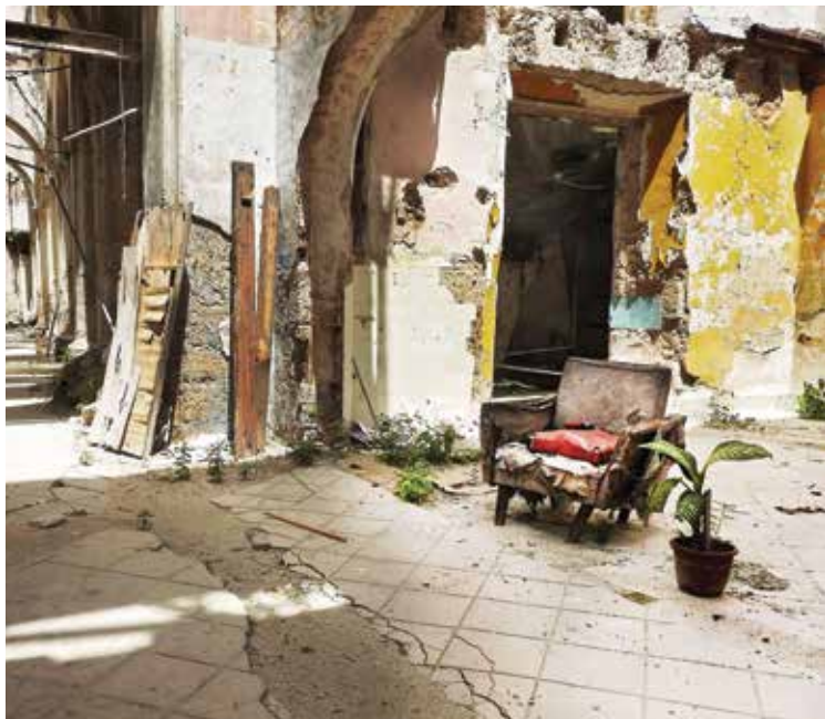
Top: Local street market in Vedado, the central business district of Havana. Bottom: Collapsed building in Old Havana.
